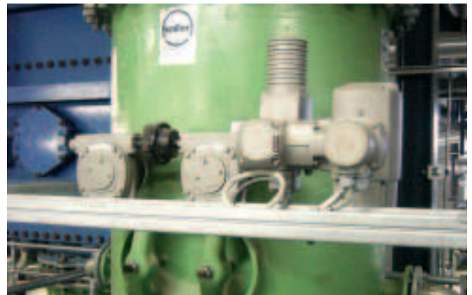
A very special solution. Two series-connected GS gearboxes are operated via one common multi-turn actuator to change the setting of a dual butterfly valve synchronously.
